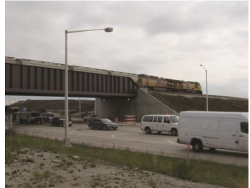
IL-19 (Irving Park Rd.) under East UP Rail Bridge
