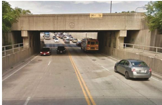
Archer Rd. Under At-grade BO-RR
